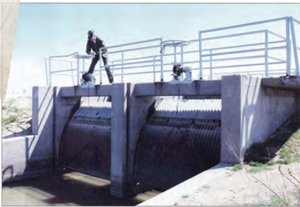
Area manager Karl Grover opens a gate, the primary means of water movement on the area.
